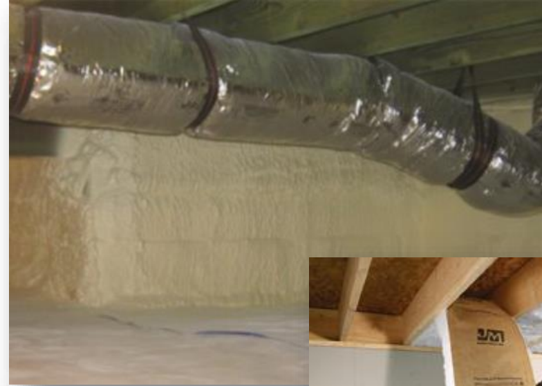
Photo from Building America Solution Center image gallery, https://basc.pnnl.gov/images
